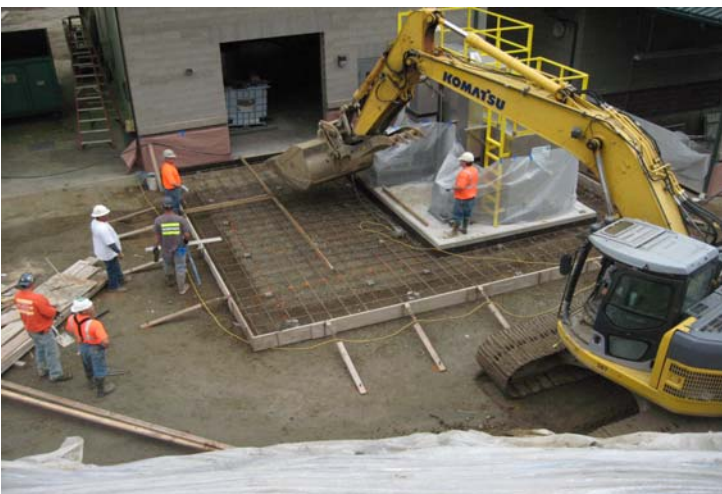
Odor Control Slab Being Completed
